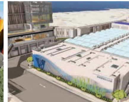
▶ Tseung Kwan O Desalination Plant (First Stage)
