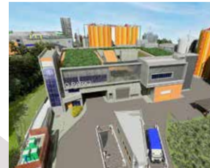
▶ Organic Waste Treatment Facilities (Phase 2)
